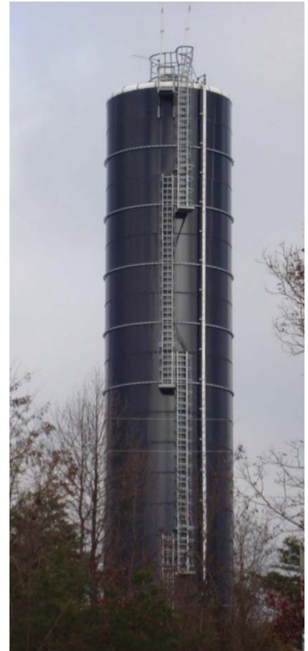
Olive Hill Water Tower
