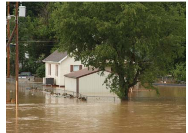
Flooding in Downtown Olive Hill
