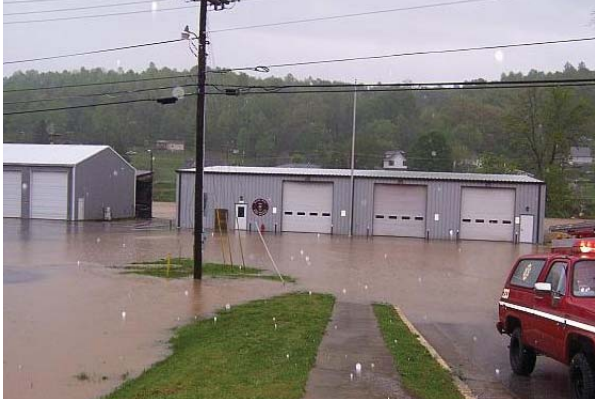
Olive Hill Maintenance Garage
