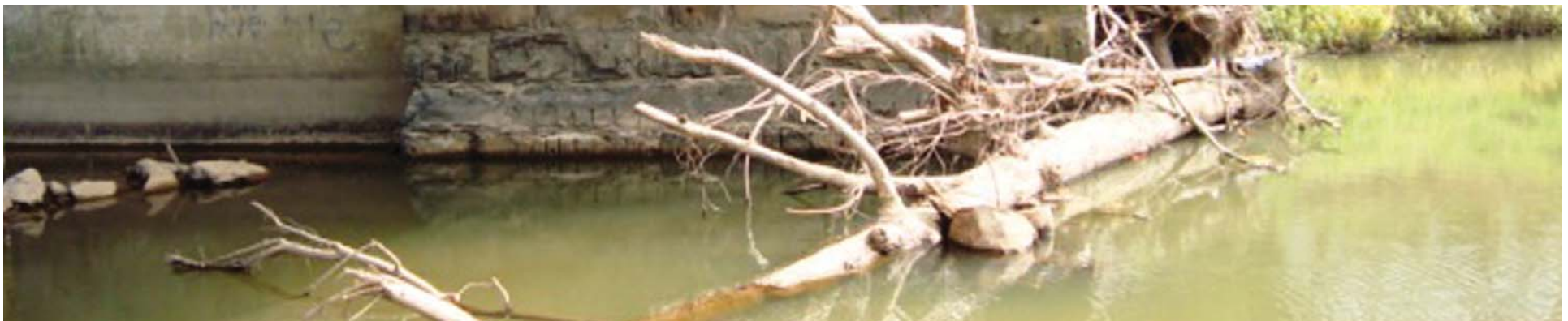
Debris left from May and July storms
