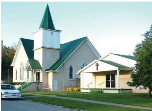
First Christian Church - Destroyed by Floods and Torn Down
